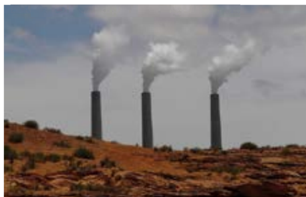
Figure 7.2 Buoyant plume rise and dispersion of stack emissions. The height of plume rise depends on the temperatures of the ambient air and the gaseous emission. For power plants and many other industries the emission is warm and will rise above the stack, thus giving an effective stack height that exceeds the actual height. (Photo credit: pixabay)
