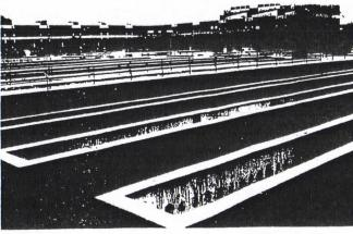
agitation causes the small clusters of suspended solids to collide with and stick to each other and form into larger particles called "flocs".
