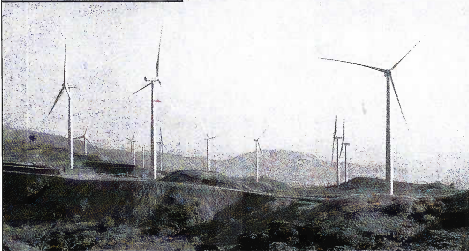
Pililla Wind Farm in Pililla, Rizal
