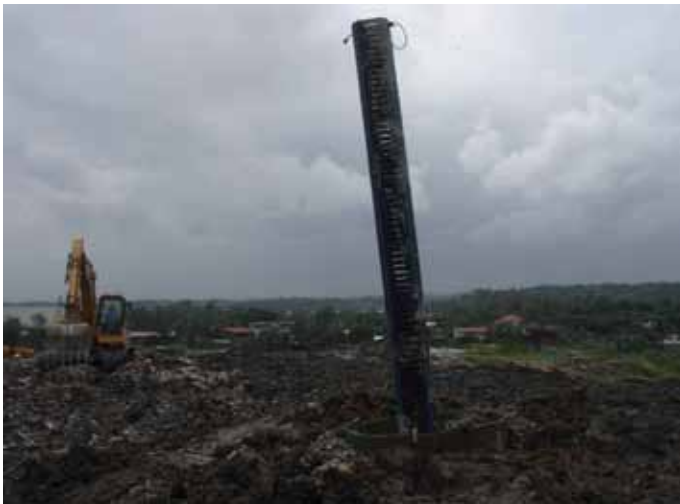
Installation of landfill gas pipes.
