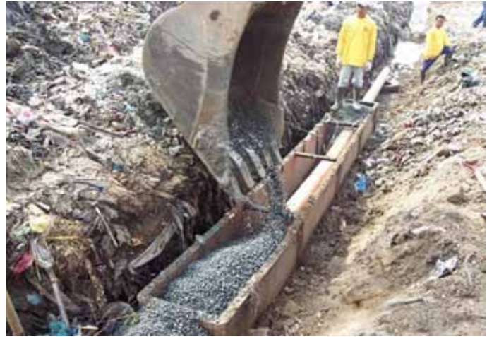
Retrofitting a perimeter leachate collector when remediating an open dump.
