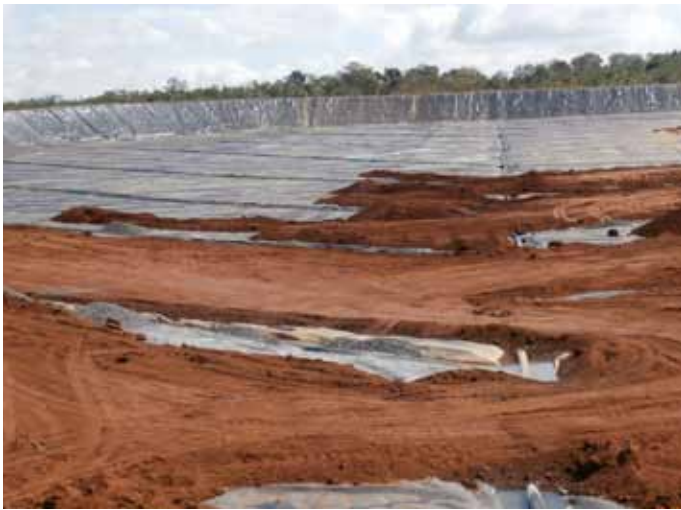
High-density polyethylene liner installation and high-density polyethylene liner damage.
