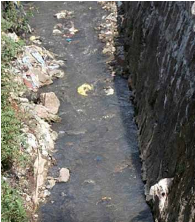
Master drainage to keep stormwater runoff out of the landfill mounds.
