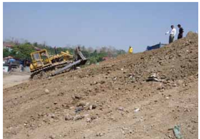
Applying soil cover material.
