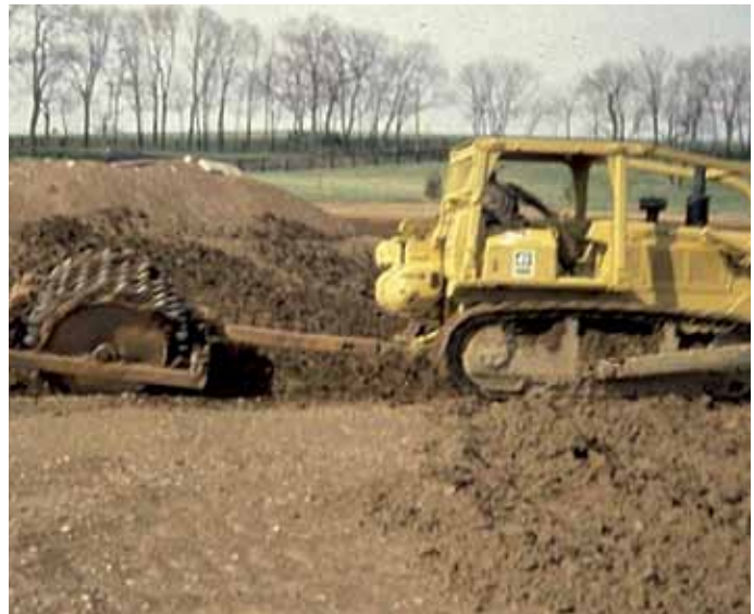
Clay liner installation.
