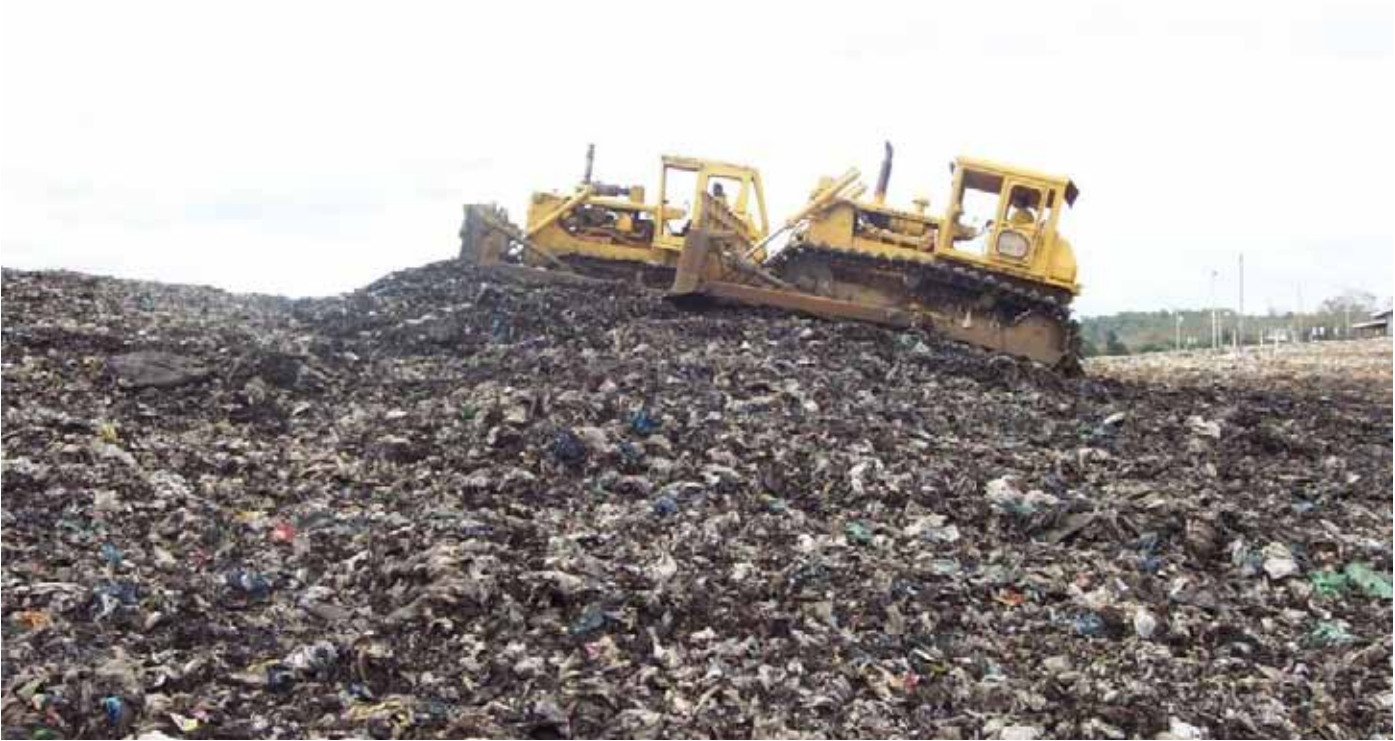
Compacting waste using bulldozers.
