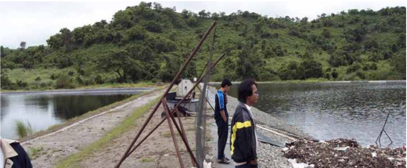
Uncovered leachate lagoon and landfill cells full after rain event.
