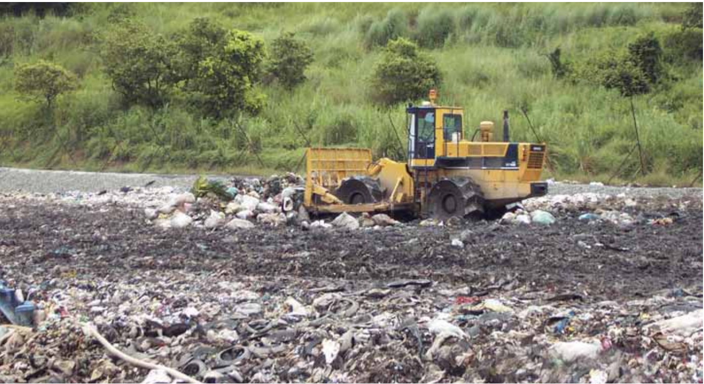
Compacting waste using a landfill compactor on a flat area.
