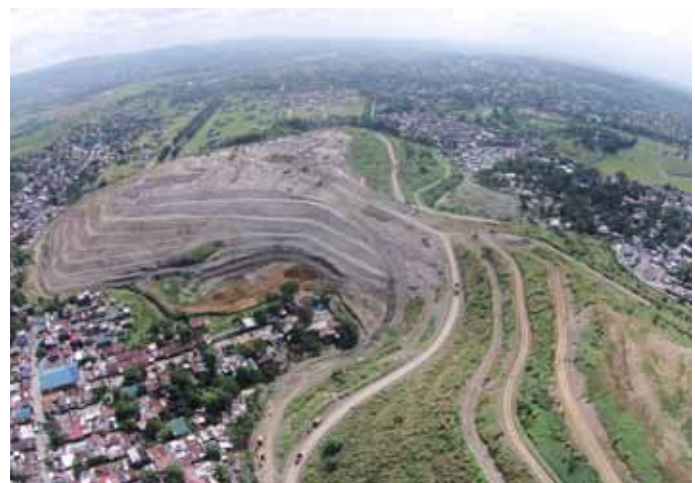
A high landfill with many lifts and benches as well as good steep external batter slopes.
