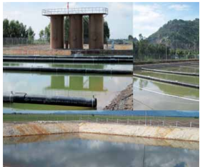
Different features of a low-technology leachate treatment plant.
