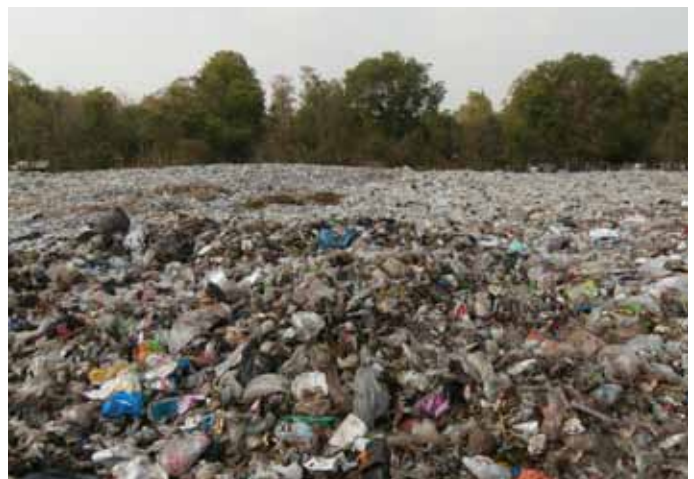
Dumpsite too flat and not covered with soil.
